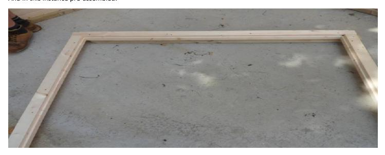
If the frame has arrived loose, the first job will be to make up the starting rectangle frame where the doors are eventually going to be hung, the frame is made up of a threshold, a Door header for the top and two uprights. These need to be screwed together with the supplied fixings, some Fitters will also like to add glue at this stage but just be sure regardless it is 100% square.
