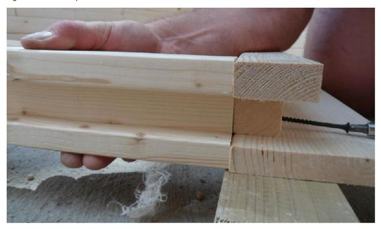
If the facia boards that create the U-Channel are not already fitted, this will be the next job as it creates a slot for the Bullnose secondary uprights to slot into later.
