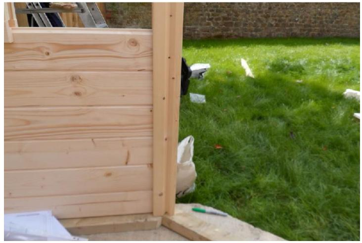
Once the Bullnose Uprights are standing in position, you can then go ahead and slot the constructed door frame into place, we have an example of how the frame slots on here to aid you with everything on the floor still. at this stage again its a good idea to check the square of the door frame.
