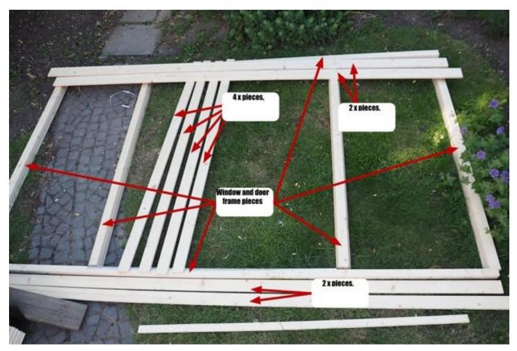
Please identify these as you are unpacking the cabin and put to one side. The door frame can be put in after the 58mm cabin has been assembled. It is easier to install if made up inside the building.
