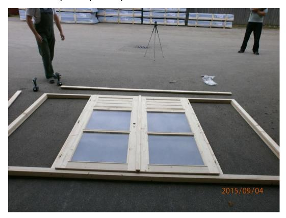
Install the side panels how you wish with screws or nails from the outside or inside. Inside hides the fittings.
