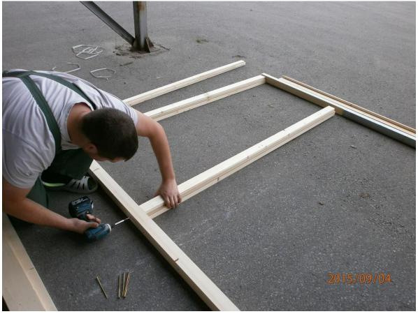
It will be obvious where the top door upright is screwed. Take a measurement of this from the side upright and transpose this to the bottom. This will ensure the centre uprights are 100% level. The metal kick plate is the bottom and maybe nipped by the door upright.
