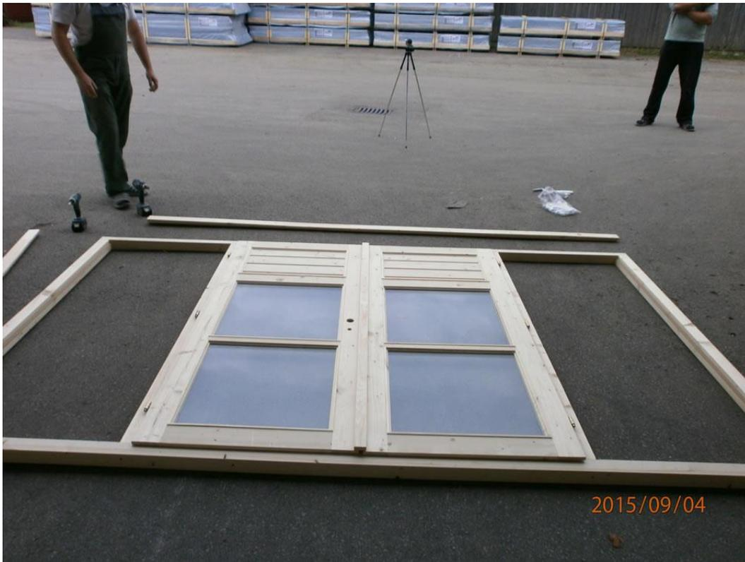
Install the side panels how you wish with screws or nails from the outside or inside. Inside hides the fittings.
